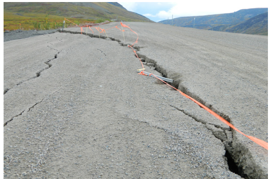
Failure of the driving surface of Dempster Highway due to melting of near-surface ground ice, km 27 in 2012.
