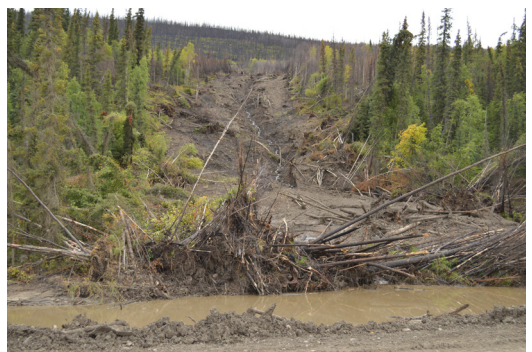
Sinkhole in 2017 at km 82 of the Dempster Highway from groundwater washing embankment materials downslope. Landslide at km 244 of Dempster Highway in 2019 after a forest fire the previous year.
