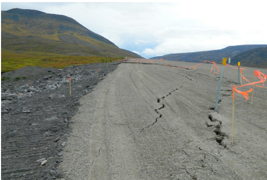
Failure of the driving surface of Dempster Highway due to melting of near-surface ground ice, km 27 in 2012.
