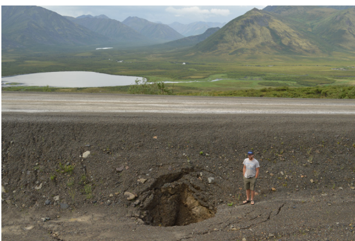
Sinkhole in 2017 at km 82 of the Dempster Highway from groundwater washing embankment materials downslope. Landslide at km 244 of Dempster Highway in 2019 after a forest fire the previous year.
